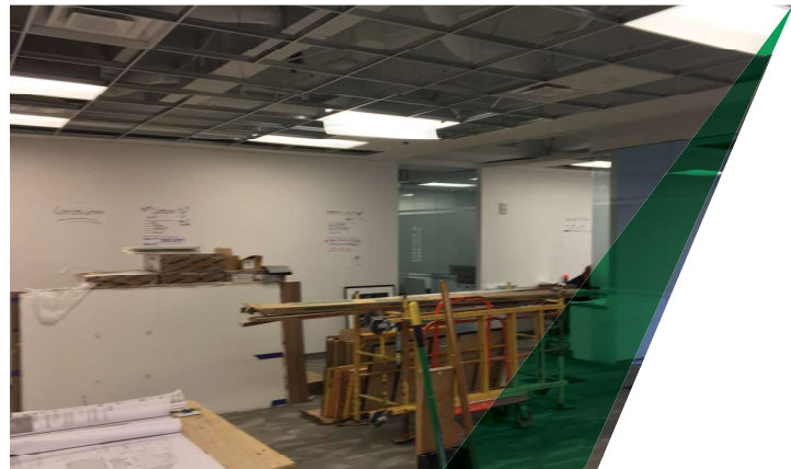
Turner Construction's Atlanta office in the midst of renovation
